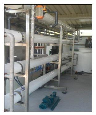
The rejected osmosis product is treated in the same process by membranes that purify this product. Two products are also obtained from this process: the filtered product, with a salt content that is treated in a second osmosis, and the rejection that will be sent to the beginning of the system or mixed with the solid fertilizer of the separation of solids.
