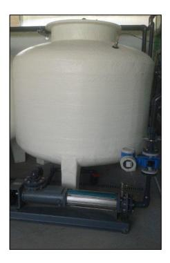
The reverse osmosis feeding tank is equipped with a pH value correction system in order to condition the product before entering the osmosis membranes.
